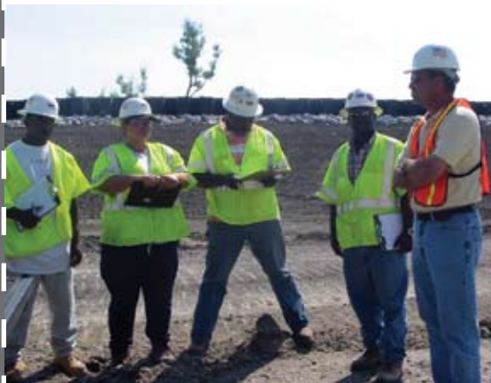
Bart Breland talks to his crew on the Port Sulphur Levee Project about the Hurricane Preparedness Plan.
