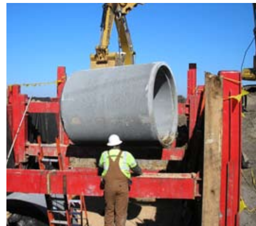
[top] Installing 72" concrete pipe across Hwy. 1088.
