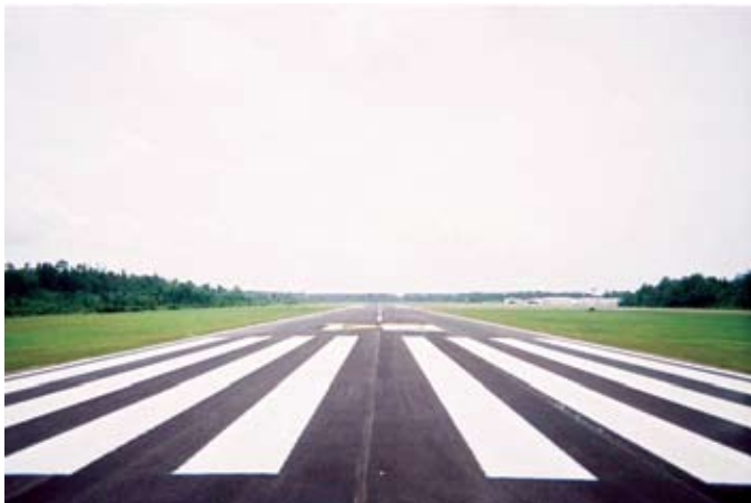
[Left] The Slidell Airport Runway project is completed. [Top] Paving the runway.
