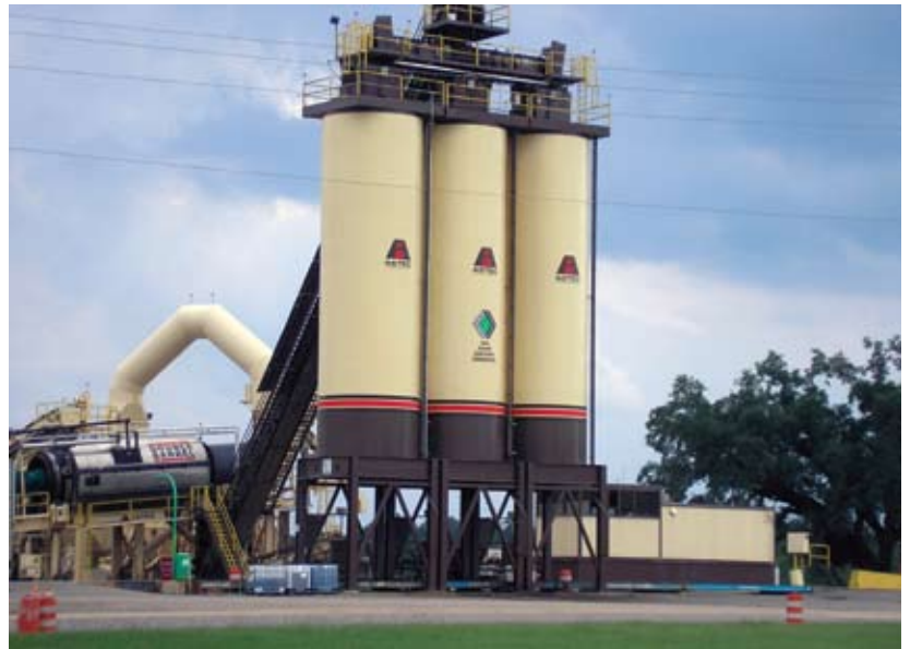
Our Franklinton asphalt plant in the morning.
