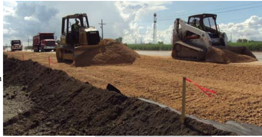
Limestone installation on the westbound side of US 61.
