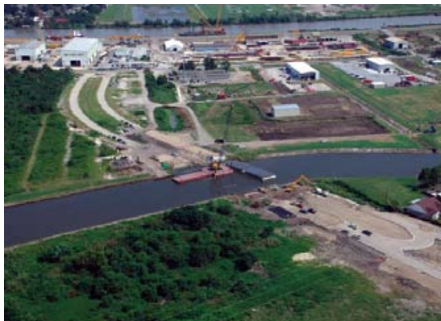
Aerial views of the Harvey Blvd. extension uniting Plaquemines & Jefferson Parishes.
