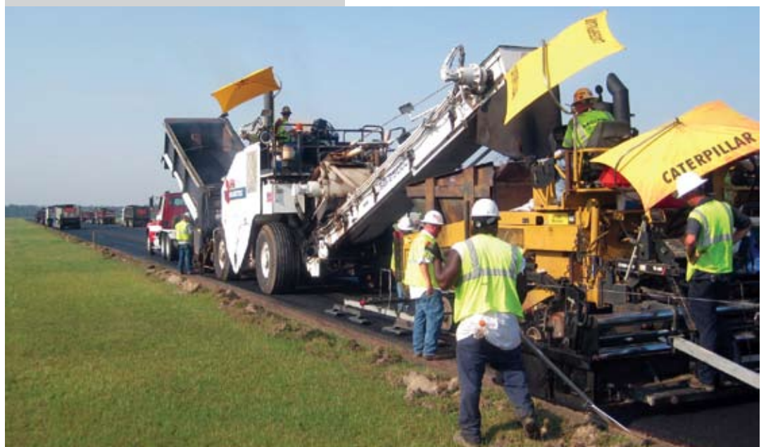
Paving the Slidell Airport Runway.
