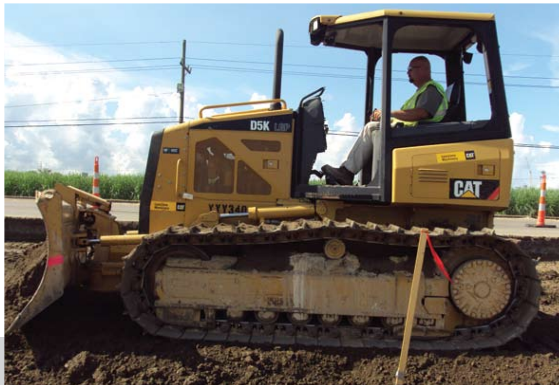
Greg Tatum, excavating the westbound shoulder of US 61.
