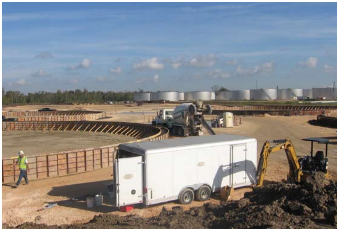
Overview of the IMTT tank terminal expansion.
