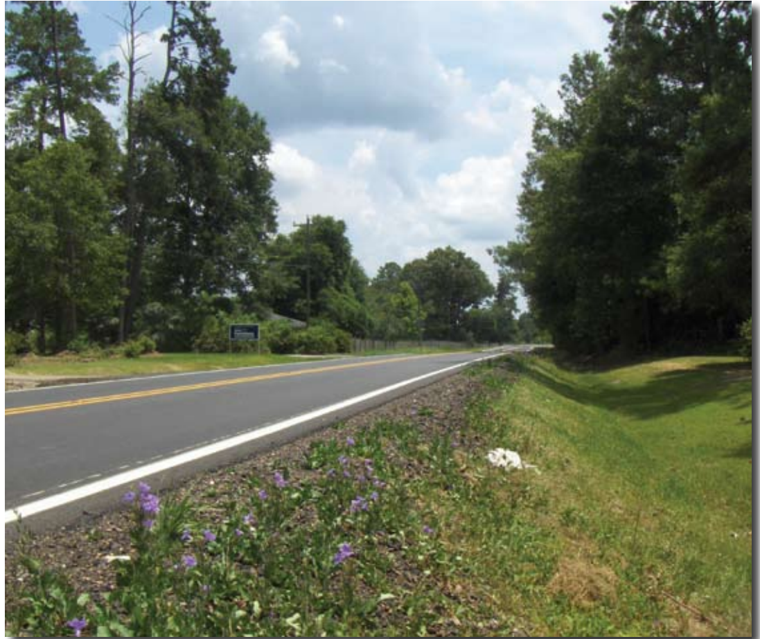
[Above and below] Purple wild flowers flank the newly-laid asphalt roadways in Livingston Parish along LA 43, as part of the DOTD projects.
