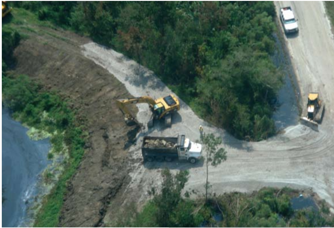
Aerial photo of the Point Celeste levee breach repairs project.
