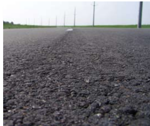
Four rollers achieved the excellent 94% compaction rate.
